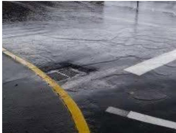
Figure 1: Stormwater draining from a parking lot
