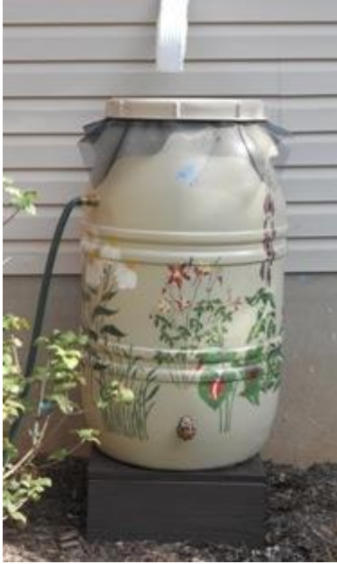
Figure 8a: Rain barrel used to disconnect a downspout with the overflow going to flower bed
